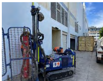
View of the drilling of in vicinity of the building footprint Inspected 17.2.2022
