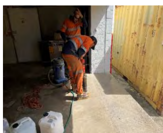
View of the concrete core at loading dock Inspected 17.2.2022
