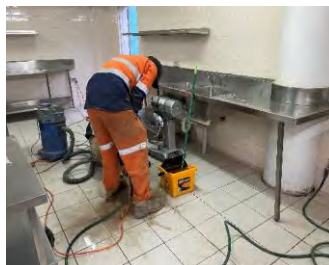
View of the concrete in side of the building Inspected 17.2.2022
