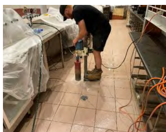
View of the concrete core in bar area, located in the centre of the building Inspected 17.2.2022
