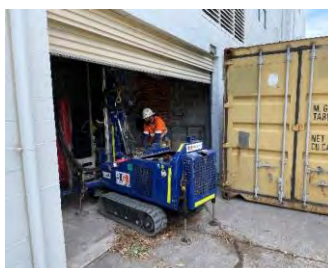
View of the drilling of loading dock Inspected 17.2.2022
